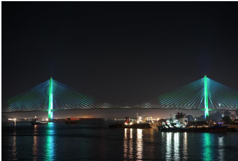
Mahkota II bridge in Samarinda, East Kalimantan, is now adorned by colorful lights, creating a beautiful crown-like view at night. This long-anticipated bridge is now the new pride of the Samarinda citizens.
