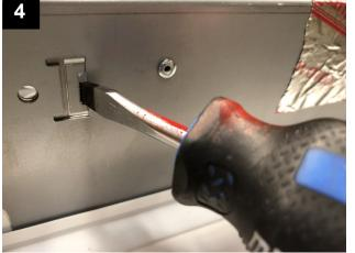
Use a flat head driver or needle nose plier to snap off the safety cover on the joiner bracket access.
