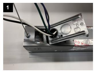
Complete power connections at wire cover. (connectors and flexible conduit by contractor) and insert inside housing as shown.
