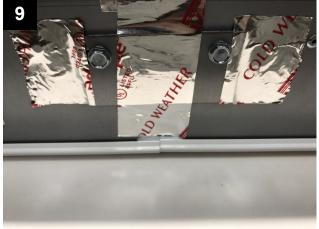
Attach and secure joiner brackets as per supplied TruGroove recessed micro drywall installation instructions.
