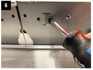
Use a flat head driver or needle nose plier to snap off the safety cover on the joiner bracket access.
