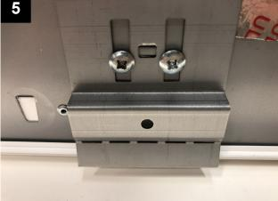
Install grid brackets at required height as described per supplied TruGroove recessed micro T-Grid installation instructions. NOTE: 4 bracket required per fixture.
