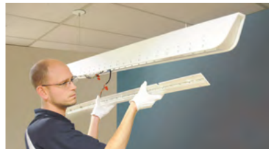
3. Remove the LED assembly.
