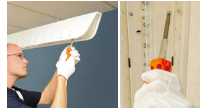
2. Unscrew the entire LED assembly from the housing.
