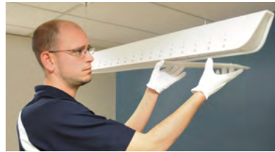
1. Lift and shift or remove the lens.
