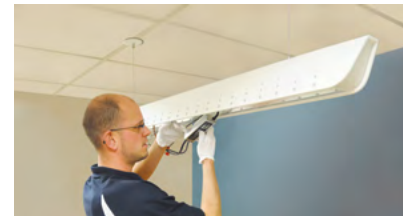
6. Remove the LED driver and replace.
