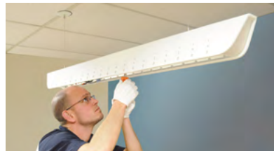
5. If required, unscrew the LED driver.
