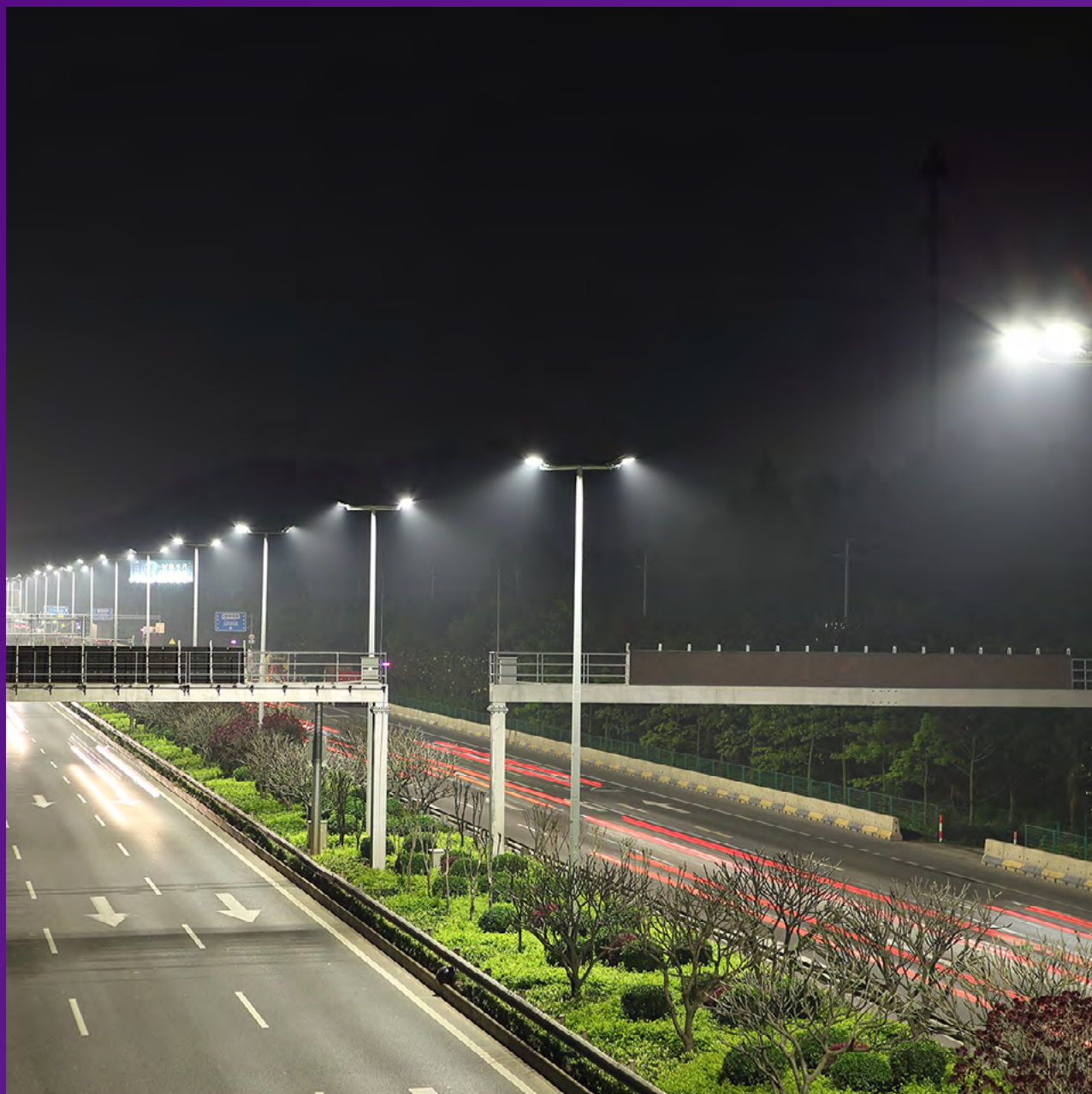
Uniform expressway lighting
