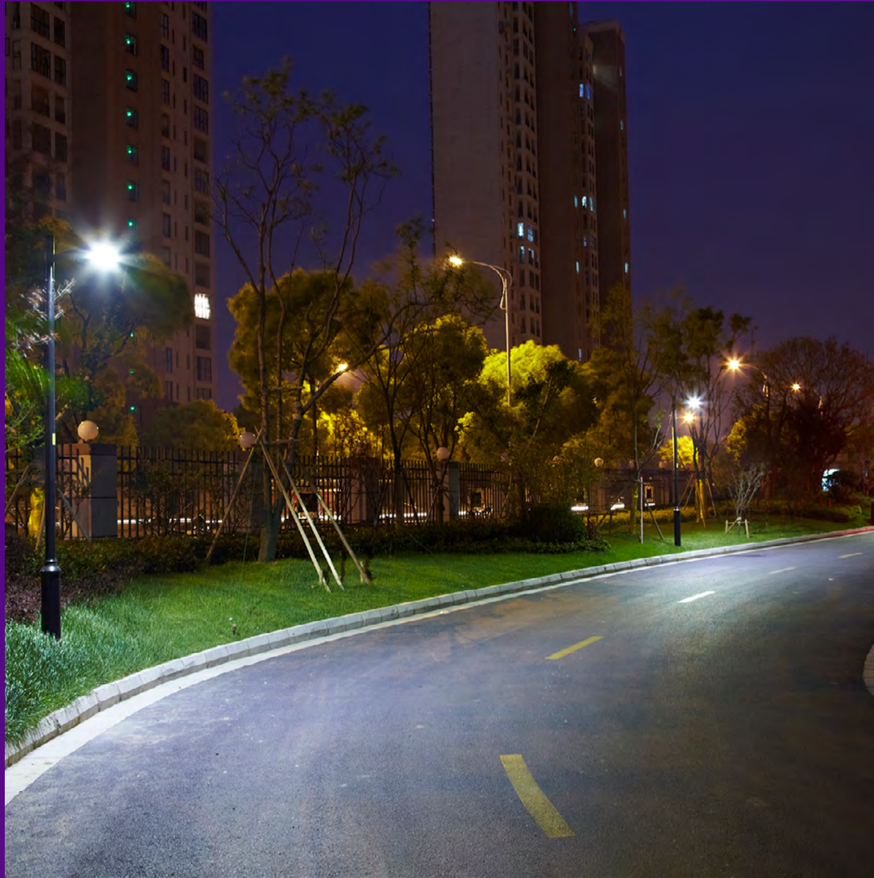
Lighting for residential and connecting roads
